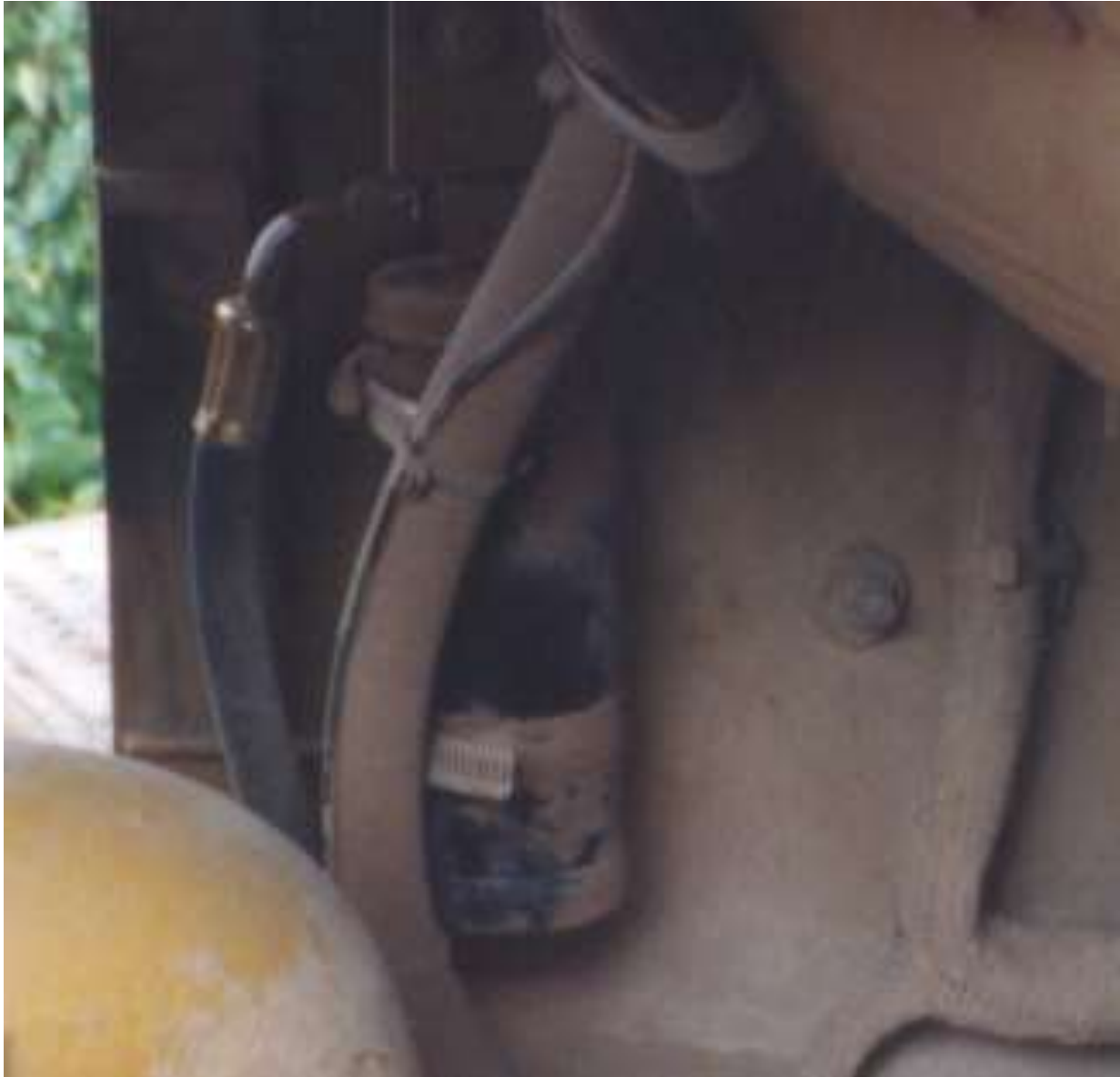
Drier in location with hoses run.
