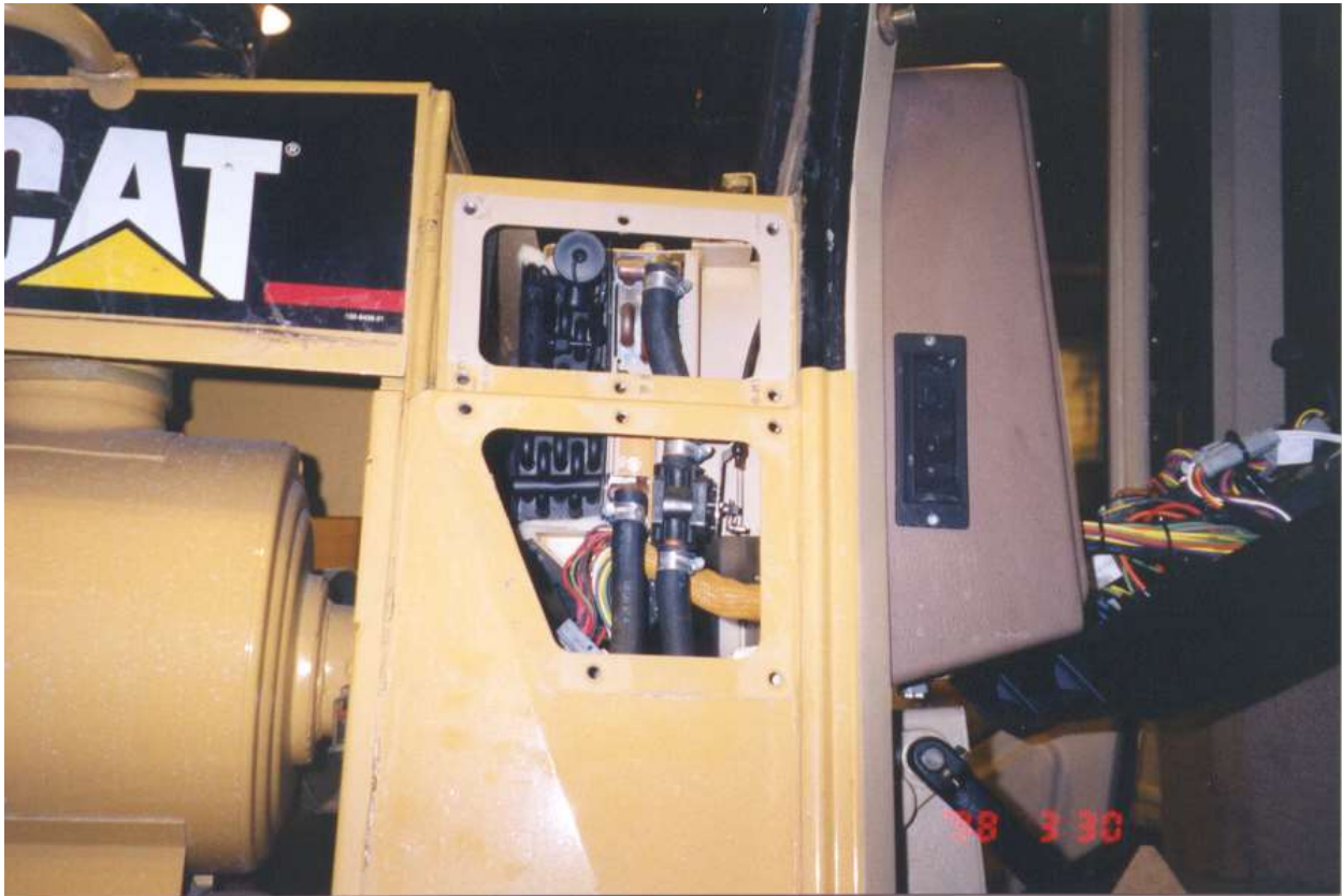
Evaporator in place alongside heater coil.
